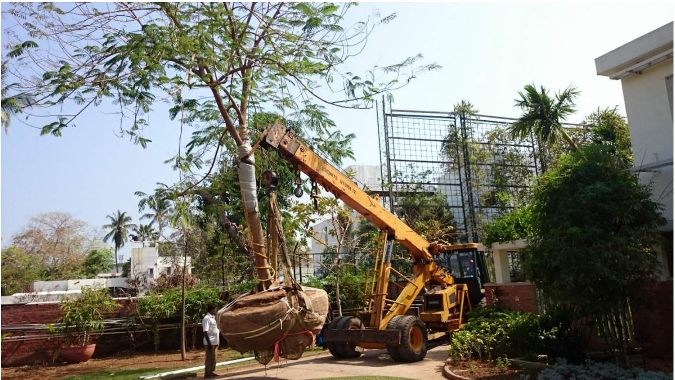
Figure 3 A crane lifting a tree in the correct manner (from the base and with protection on the stem in case of knocking)
