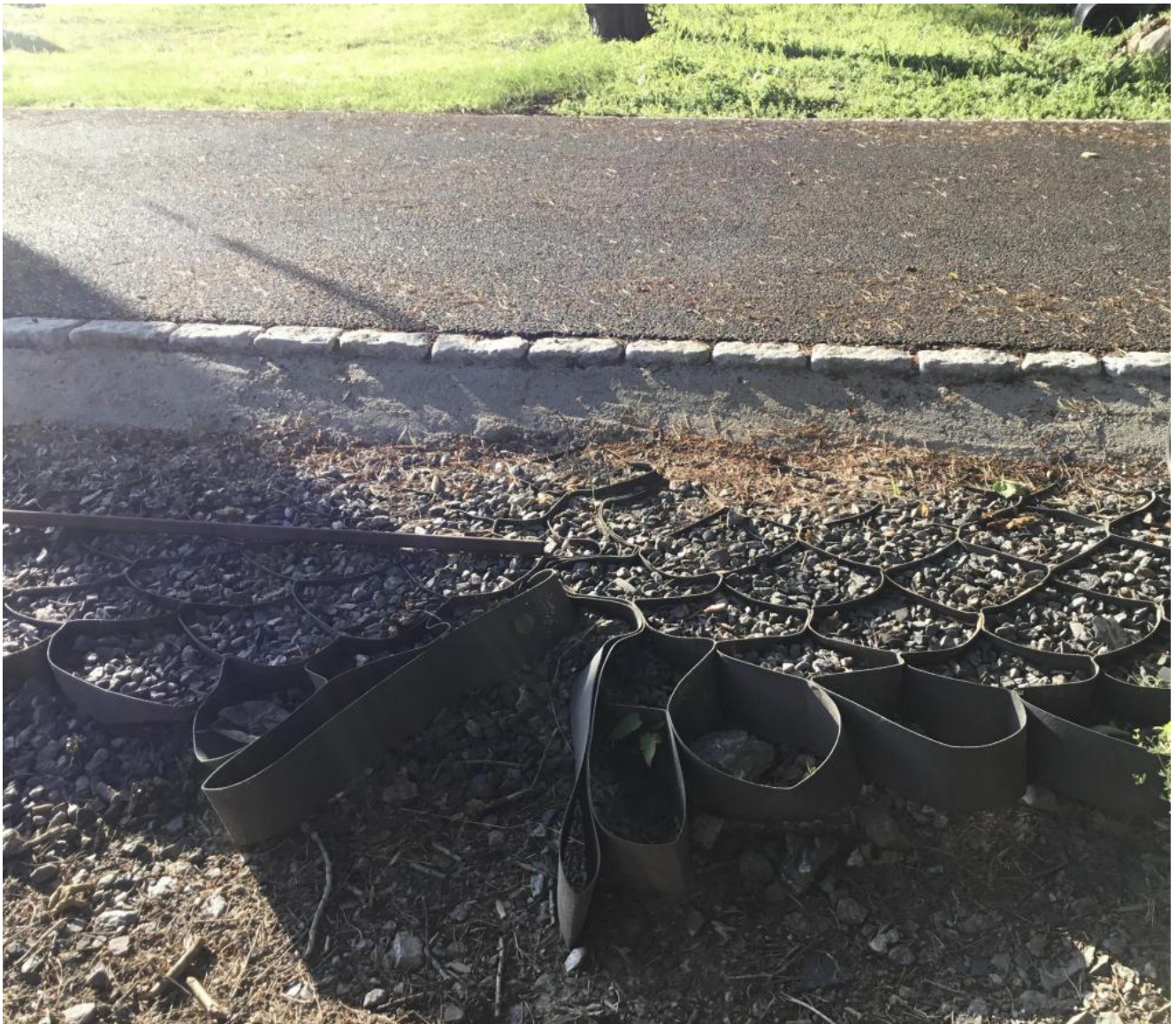
Figure 5: Example of permanent tarmac using Geowebb or similar. Exposed Geowebb is only there to show that it is present but would normally be covered/under the road.
