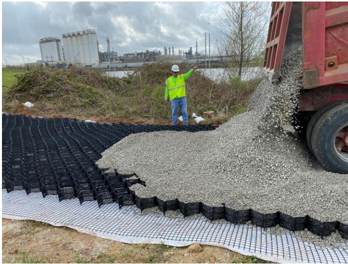
Figures 3 and 4: Examples of Geocell technology (available in India)
