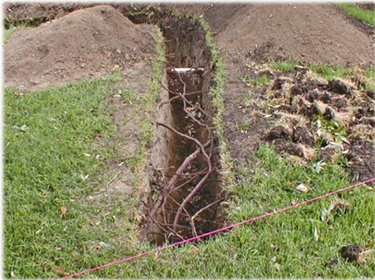
Figure 7: The result after using a pneumatic excavator.
